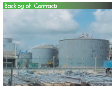
• Blasting tank in progress
